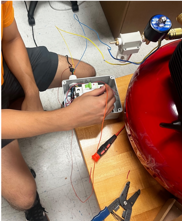
Figure 19: Sampler Bleeder Controller Fabrication
